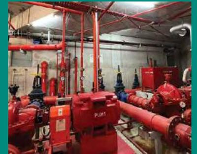
**In support of our tenant, we completed a water saving project at 4 Pandan Avenue, Singapore in January 2023. This project involved the upgrade of the sprinkler pipeline and installation of a pressure relief valve that enabled the recycling of water which would otherwise have been drained off during the weekly sprinkler system testing. This project resulted in an estimated 80% reduction (2,900 CuM) in water consumption which translates to S\$7,950 in savings annually<sup>16</sup>.**
